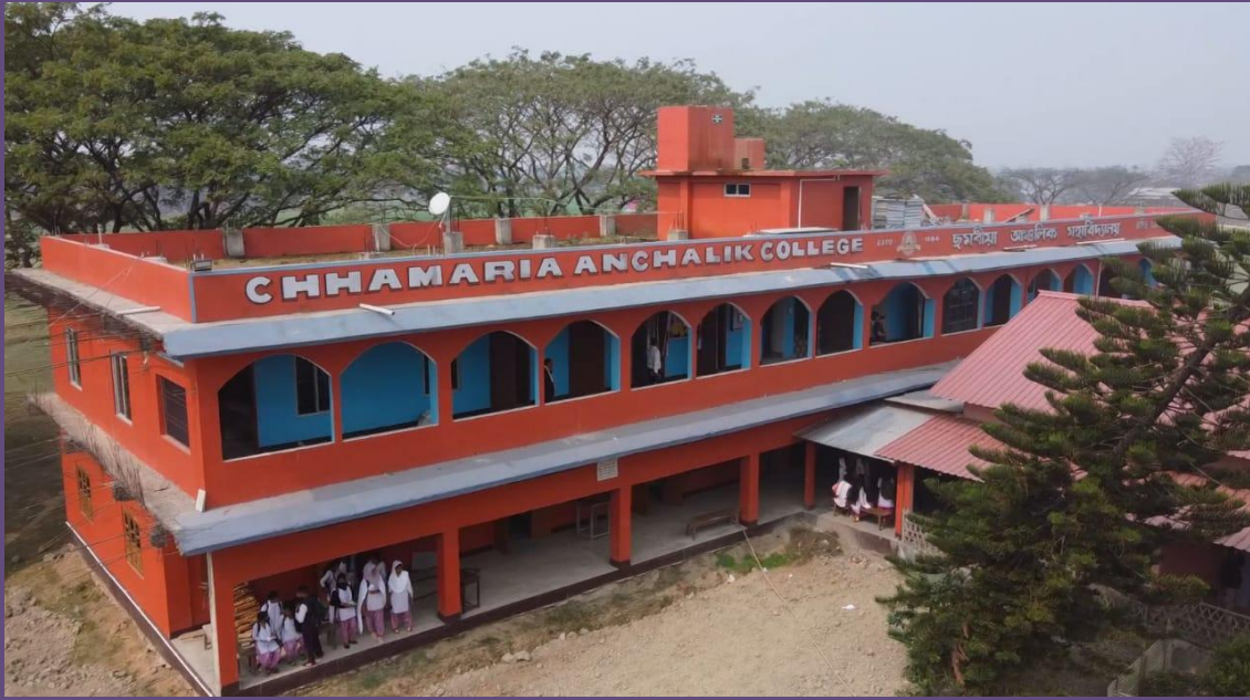
R.C.C TWO STORAGE COLLEGE BUILDING
